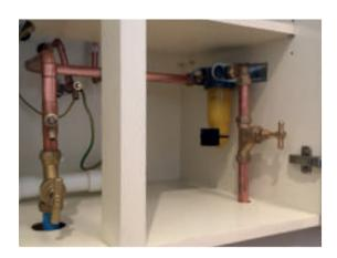
Standard installation example of a CombiCompact unit to a main incoming water supply to a dwelling under sink installation
